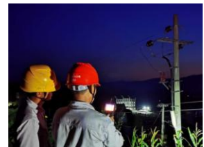
Electrical Equipment Monitoring
